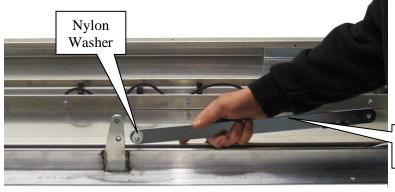
**3.** Install a nylon washer on the stud on the end of the Straight Linkage.
